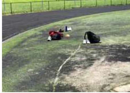
THIS FIELD HAS SUBSEQUENTLY BEEN REPLACED. THE SAND IN BOTH PHOTOS HAS RUN IN FROM THE TRACK AND FIELD PIT.
