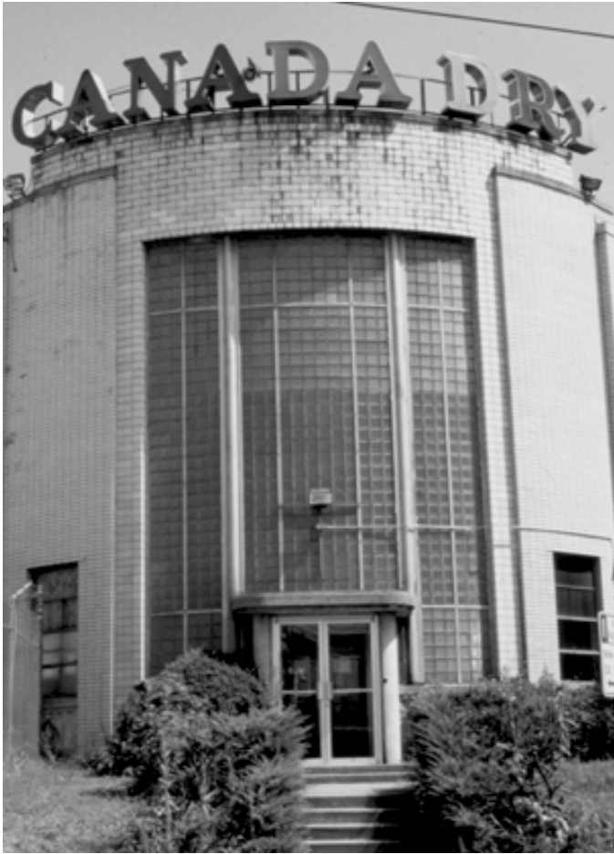
Canada Dry Building in Silver Spring —Photo provided by Mary Reardon
