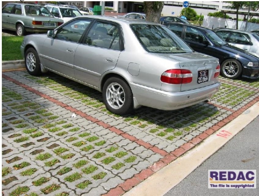
Figure 4 - Porous Driveways and Parking Areas
