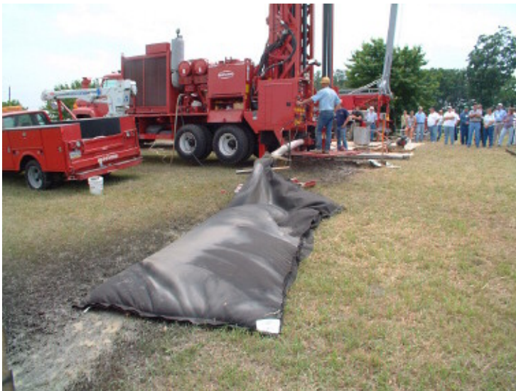
Figure 6 - Dewatering using Filtering Bag
