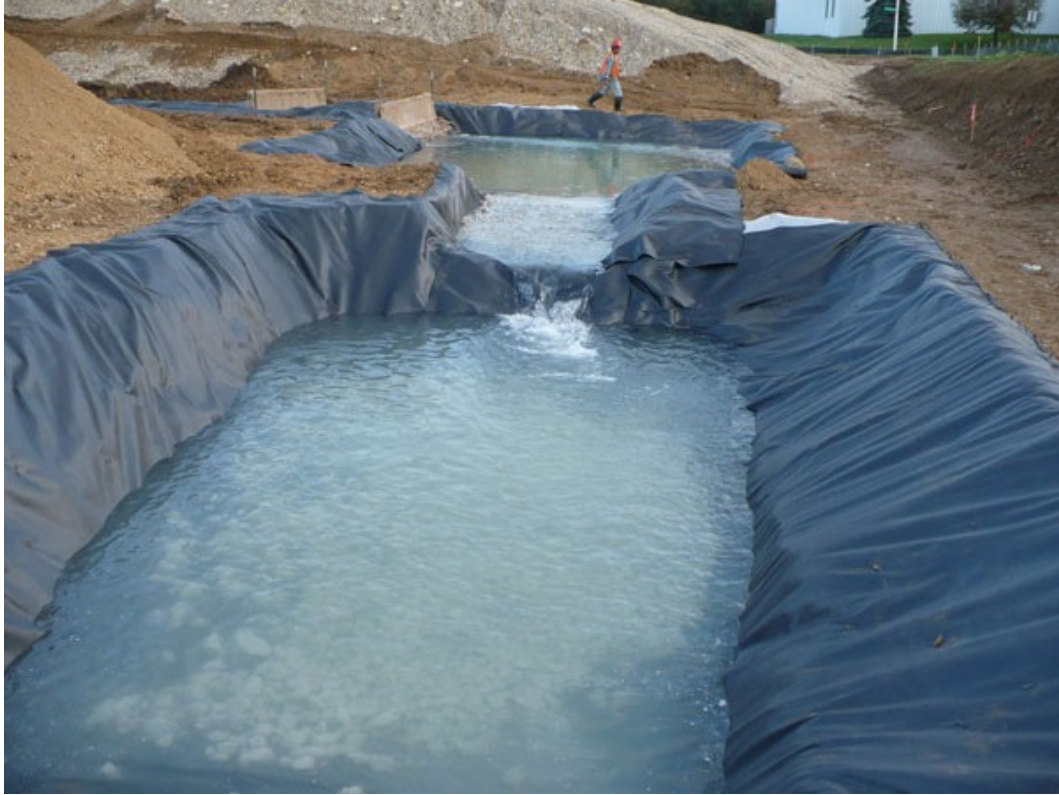
Figure 5 - Maintenance & Dewatering of Traps using Filtering Cloth
